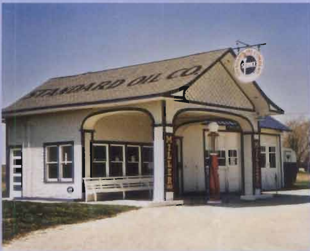
This 1932 Standard Oil Filling Station, located on the original Route 66 in Odell, IL, was purchased by the town and restored by Odell Tourism and Community Development Board, the Route 66 Preservation Committee of Illinois and many other volunteers and contributors. It functions as a museum and visitor center. Photo: John and Lenore Weiss and the Route 66 Preservation Committee of Illinois.
