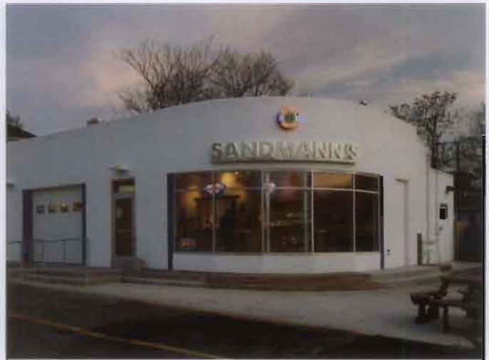
Figure 15. The historic restroom door to the right of the display window was closed off (and entry provided on the inside) when this former gas station in Grand Rapids, MI was converted to a carry-out restaurant. A flush panel was recessed in the opening to identify the historic location of the door. Photo: M Buck Studios.
